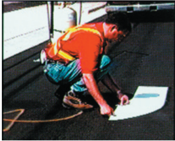
Figure 5.2 Placement of material
