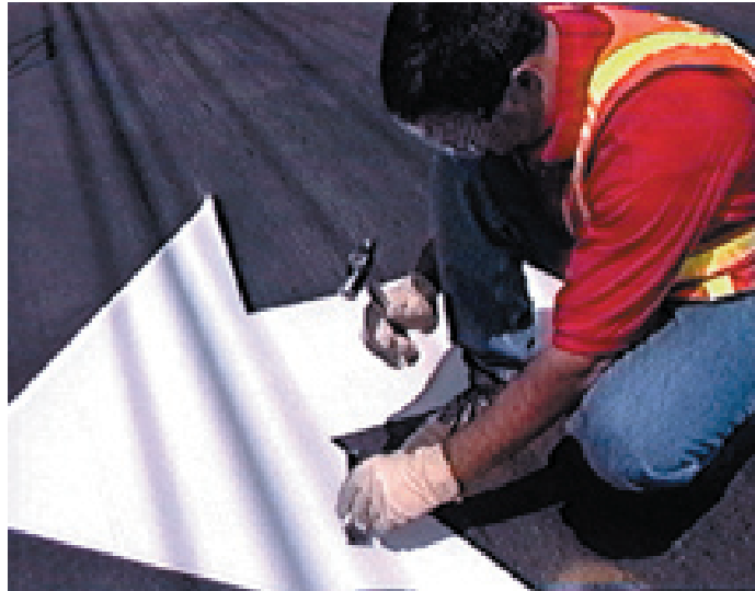
Figure 5.4 Adhesion test being performed
