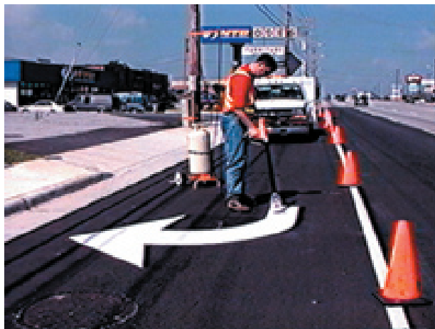
Figure 5.3 Arrow symbol being applied by heat torch.
