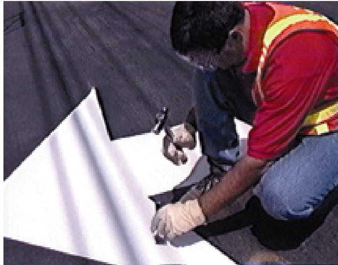
Figure 5.4 Adhesion test being performed
