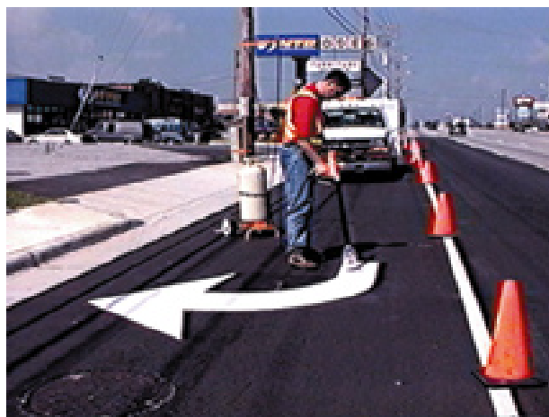
Figure 5.3 Arrow symbol being applied by heat torch.
