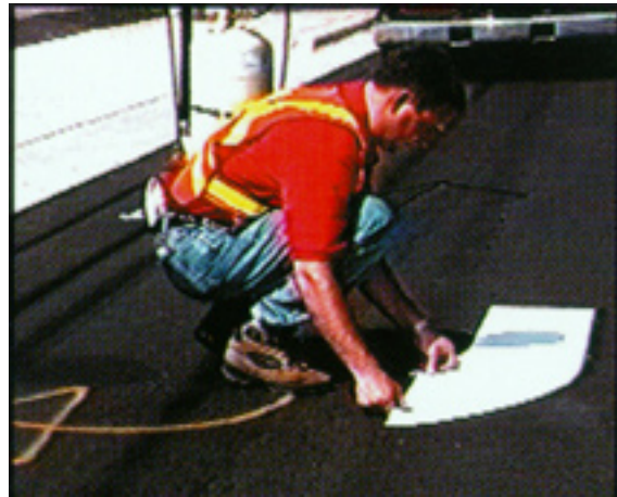
Figure 5.2 Placement of material
