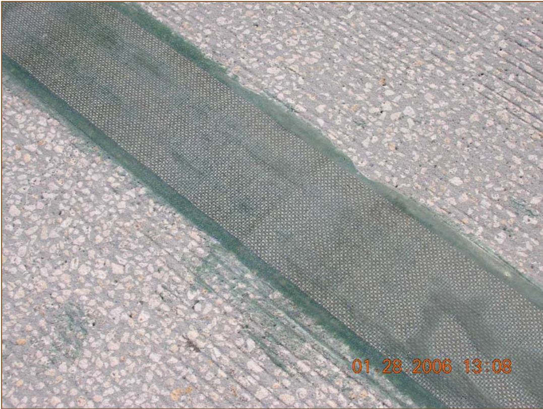
Figure 7 Carbon fiber mesh repair.
