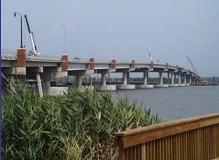
Rte. 33 over the Mattaponi River at West Point, Virginia
