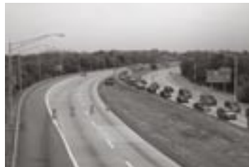
Virginia prepared for hurricanes with a Hurricane Evacuation Route Analysis and an upgraded lane-reversal plan. (Artist's rendering, at left).
