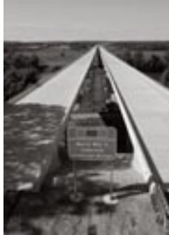
Route 288: PPTA finished in 2004.
