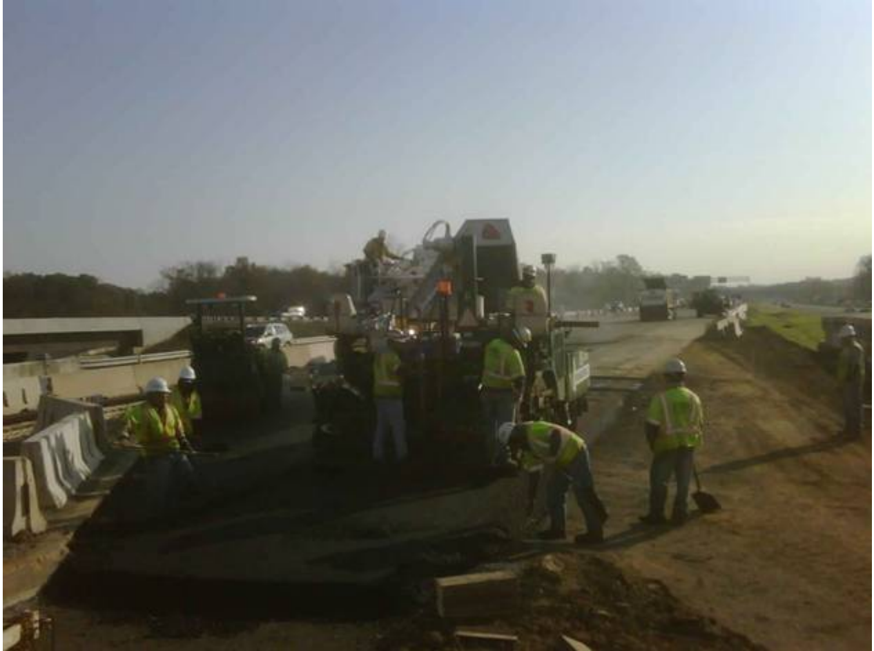
I-66 Westbound – Placing intermediate asphalt on westbound lanes.
