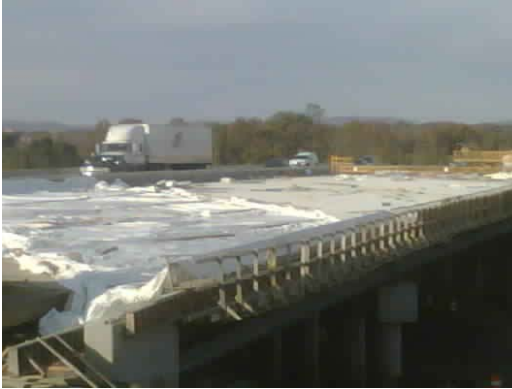
B629 – Finish placement of all five deck pours (eastbound).
