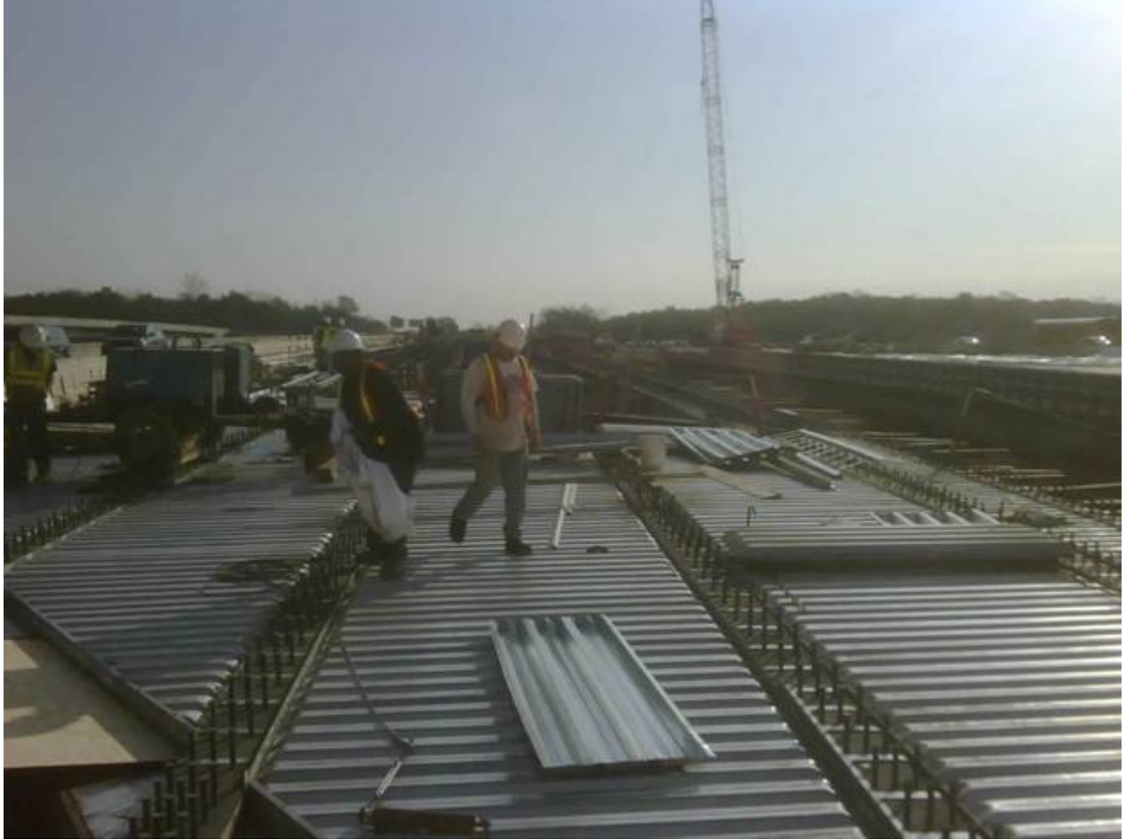
B630 – Installation of deck pans
