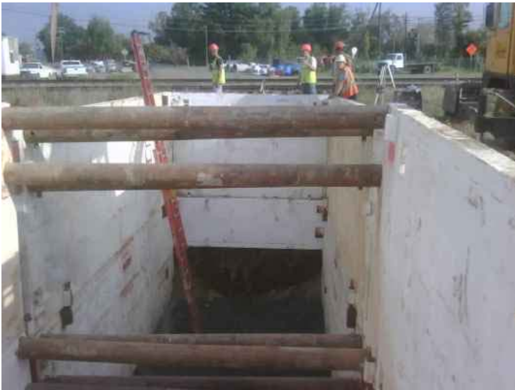
Jacking Pit for 24 inch bore under the Railroad
