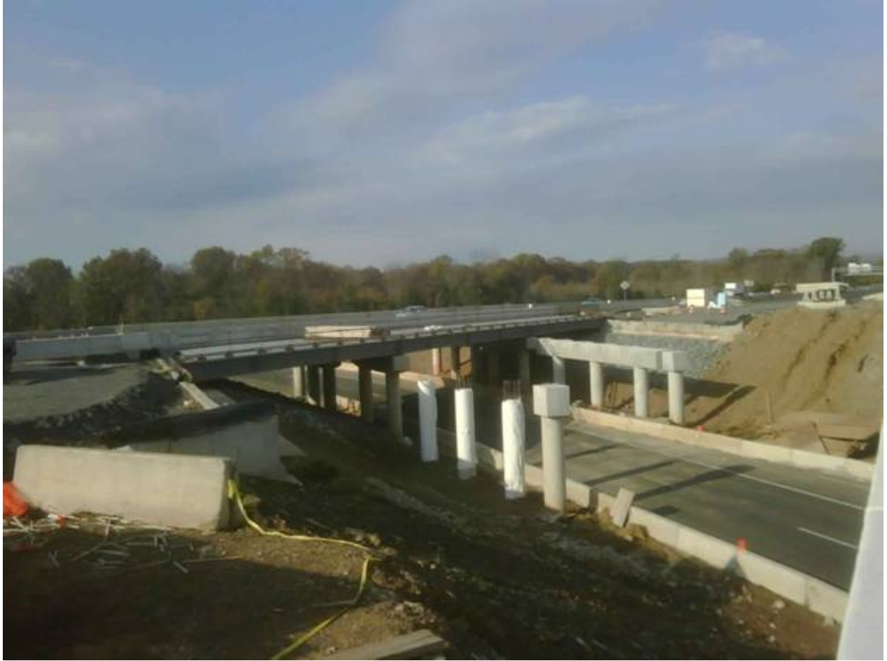
B627 – Finish pier column on Pier 2 and Pier 1 pier cap.
