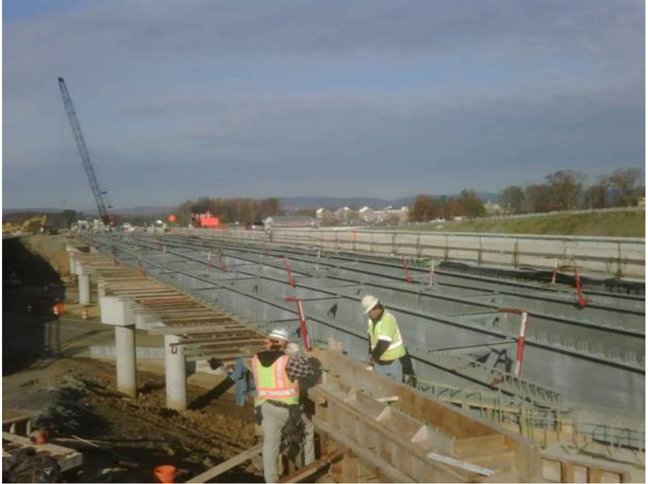
B630 – Installation of parapet formwork.
