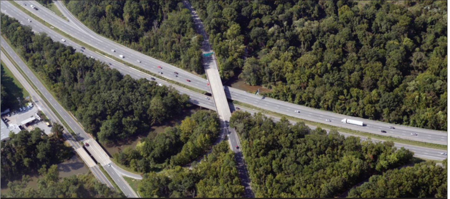
Upham Brook Bridge Overpass, I-95, Richmond, VA (Photo by VDOT)
