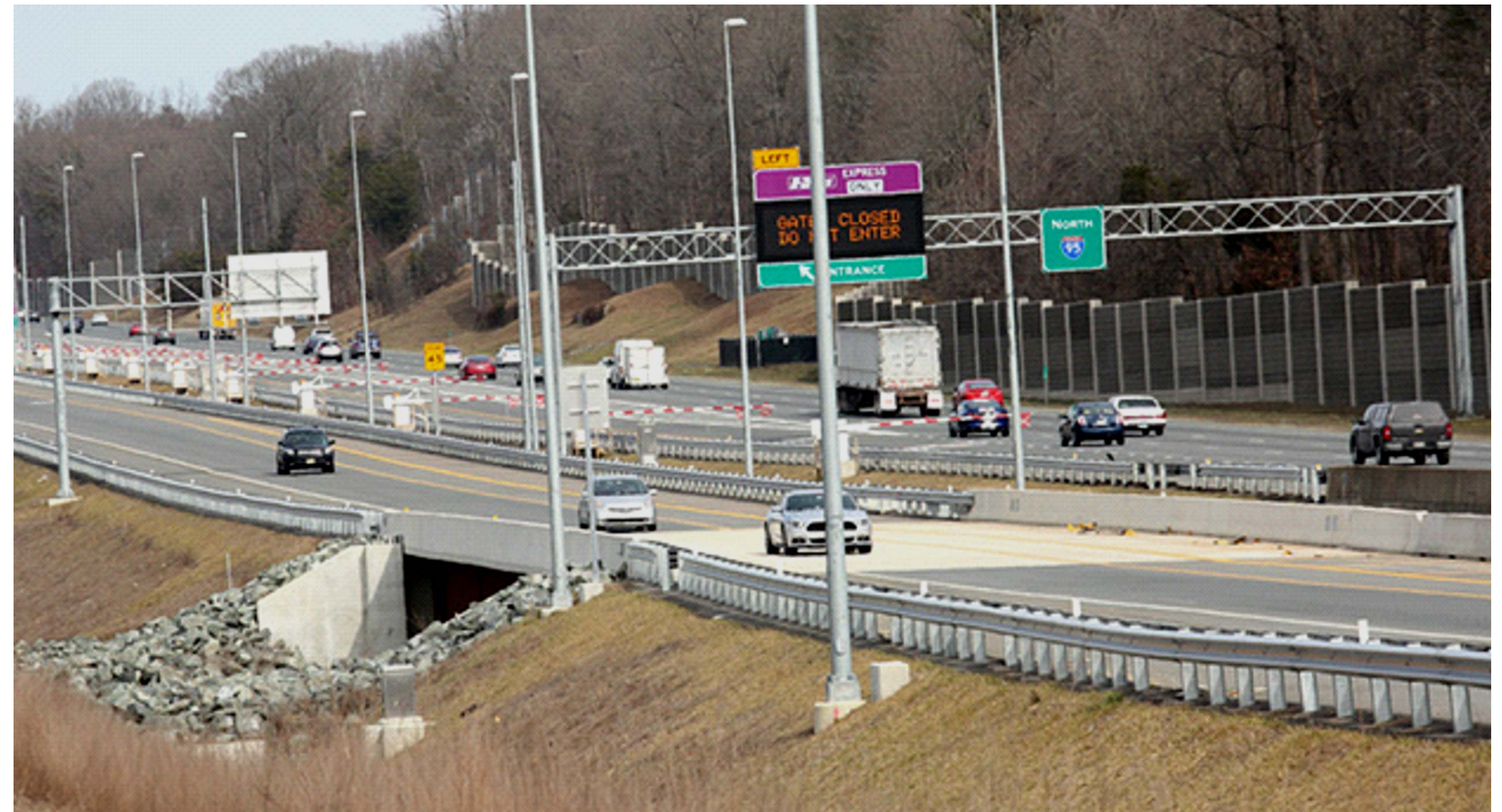
Photo: I-95 HOT Lanes in NOVA
