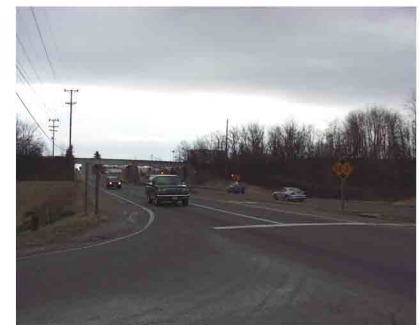
Field photo from Bagging Plant Road center line looking south along Route 100.
