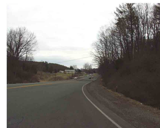
Field photo of existing intersection of Old Route 11 and Route 11. View of photo is to the east from the center of Old Route 11 exit lane.
