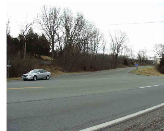
Field photo of existing intersection of Old Route 11 and Route 11. View of photo is south-west from opposite side of roadway.
