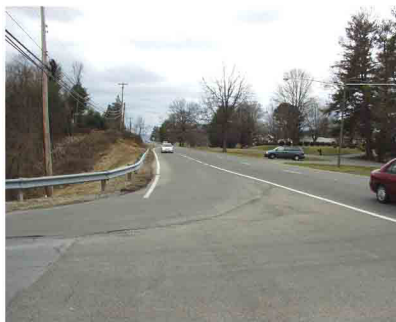
Field photo of existing intersection of the Hospital Entrance and Route 11. View of photo is to the west from the exiting lane of the Hospital Entrance.
