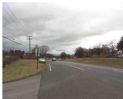
Field photo of existing intersection of Hatcher Road and Route 11. View of photo is to the west from the center of Hatcher Road exit lane.
