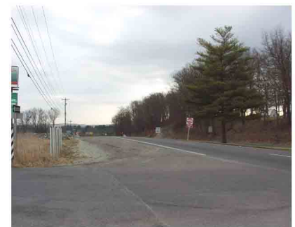
Field photo of existing intersection of Roundhouse Road and Route 11. View of photo is to the east from the center of Roundhouse Road exit lane.
