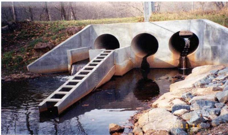
**Figure 9. Steep pass design for Claiborne Run. Note adjustable gated flow wall to left of steep pass structure.**
