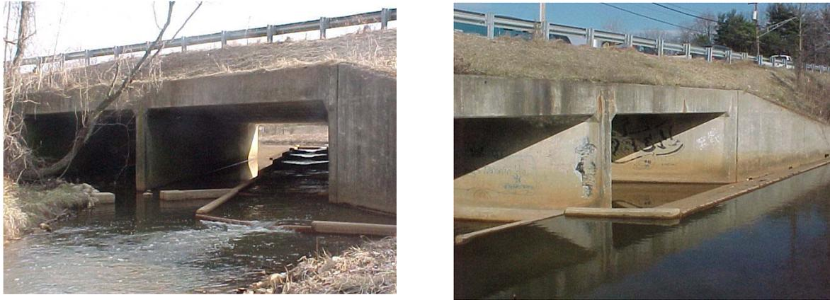
Figure 5. Sawmill Creek culvert and downstream and upstream views of the custom pool-weir fish passage.
