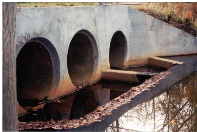
**Figure 10. Upstream diversion wall for fish passage system. Wall to right of picture has removable gates that are presently keeping water level even through the three pipes. Removable gates make maintenance and flood control easier when passage is not required.**
