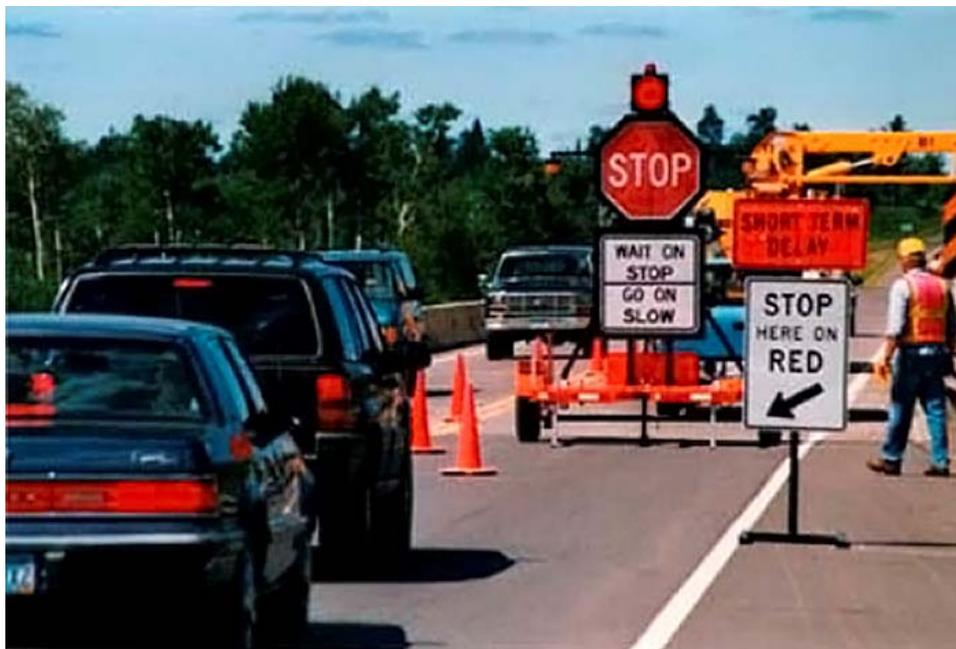
Figure 1. AutoFlagger. Source: <http://www.AutoFlagger.com/AutoFlagger.htm>. Reprinted with permission.
