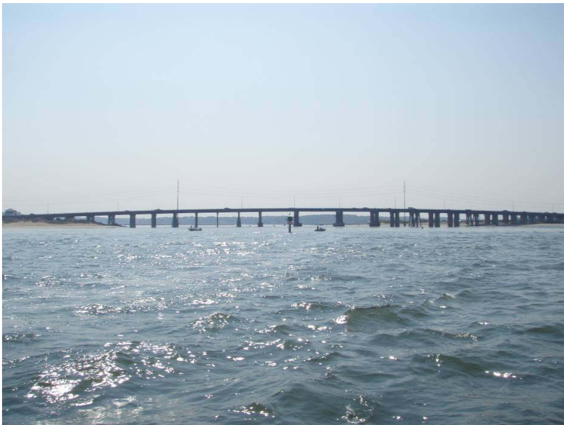
Figure 2. North Elevation of Lynnhaven Bridge 5
