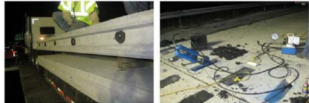
**Prestressed precast concrete pavement system**
