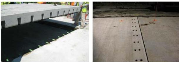
**Precast concrete pavement system**
