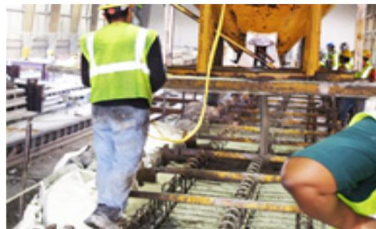
**Placement of self-consolidating concrete into beam at the plant**
