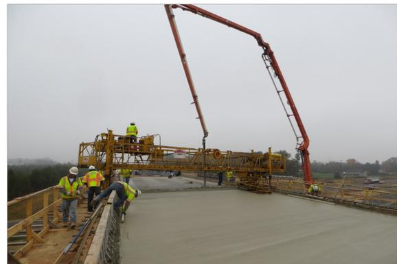
**The lightweight high-performance concrete deck on the U.S. 17 flyover interchange bridge has weathered three winters with no cracks detected.**
