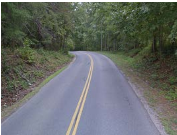
Sample road segment with centerline markings only
