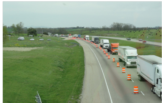
Innovative traffic management routes passenger vehicles to a primary road and channels trucks through the work zone in one lane.
