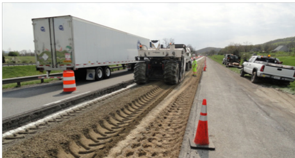
Full-depth reclamation mixes base aggregates and soil with stabilizing additives.
