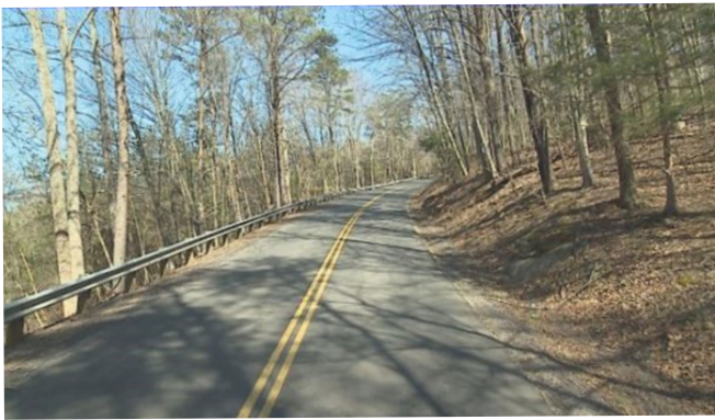
Guardrail shields an embankment slope on a low-volume Virginia rural road. (VDOT i-vision image)
