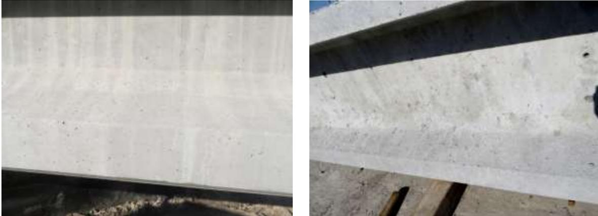
**Figure 2. Surface of SCC (left) and of Conventional Concrete (right)**
