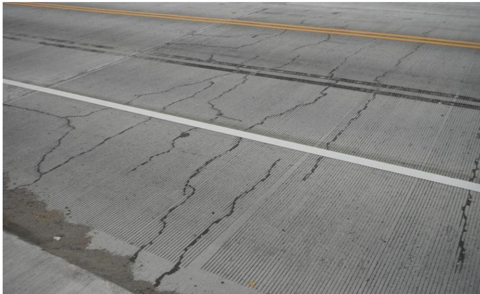
**Figure 3. Transverse Cracks on Route 61 Over New River (Salem District)**
