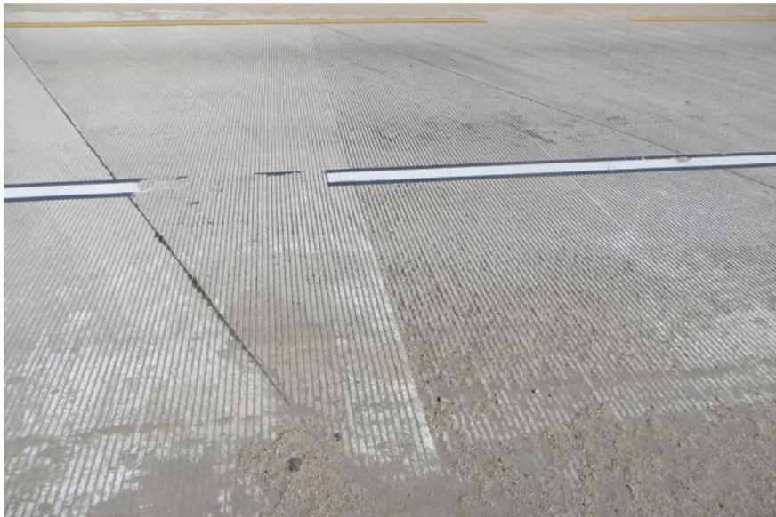
**Figure 7. Scaling at Closure Pour of Route 15 Opal Bridge at Lower Middle Portion of Photograph**
