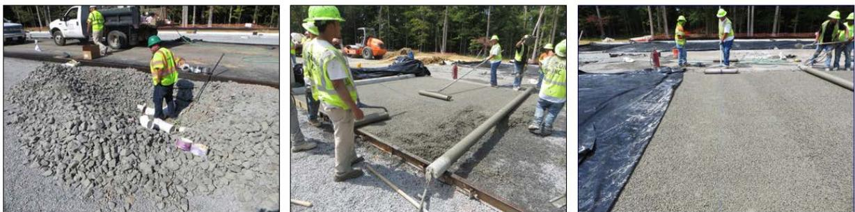
**Figure 1. Construction Sequence at the Stringfellow Lot (L-R: Perforated Pipe Being Placed in the Loose Aggregate; Two-Directions of Rolling Compaction; Joints Being Placed)**
