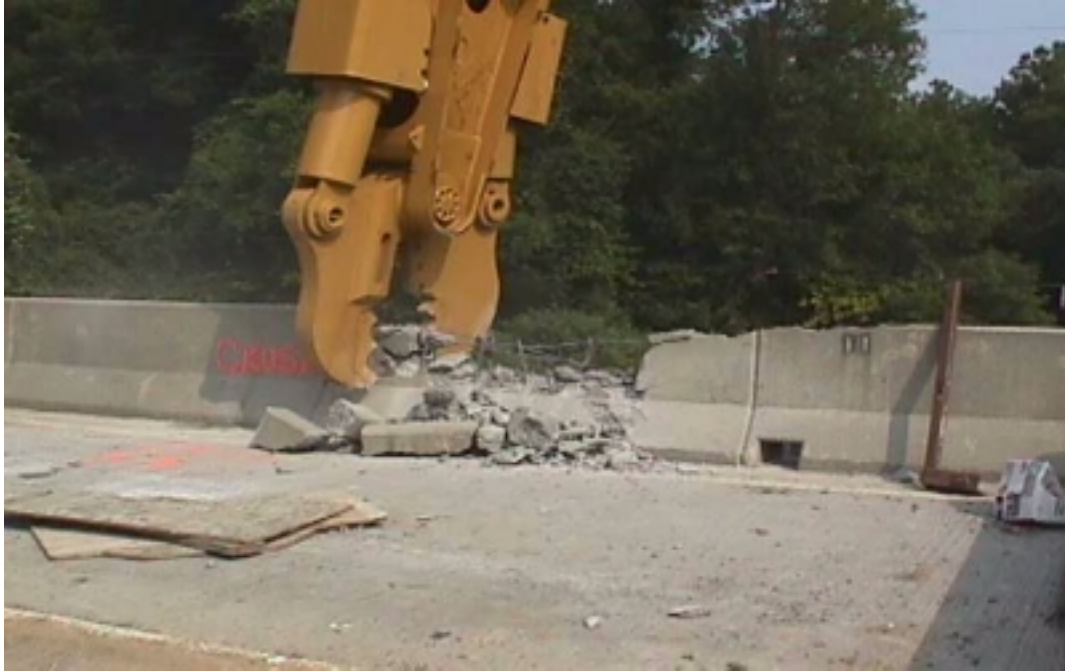
Figure 6. Concrete Removed Using Concrete Crusher
