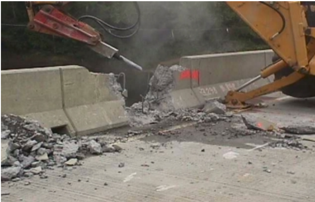
Figure 5. Parapet Demolished Using Hoe Ram
