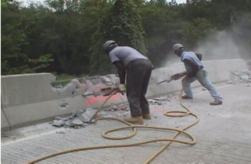
Figure 4. Concrete Removed From Parapet Using 90-lb Hammers
