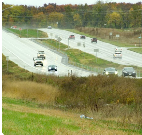
Boone County, MO RCUT Intersection Source: RCUT Video FHWA-SA-14-020
