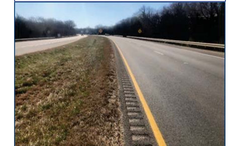
Edgeline Rumble Strips
