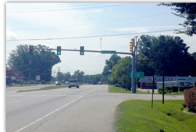
Route 17 looking southbound at Brick Church Road
