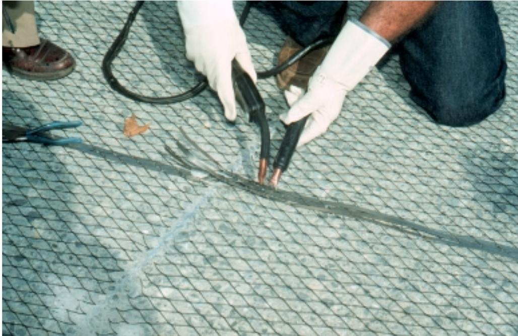
**Figure 3. Electrical bonding of all anode mesh by resistance welding to several strips of titanium ribbons, which were subsequently connected through lead wires to the positive terminal of the rectifier.**
