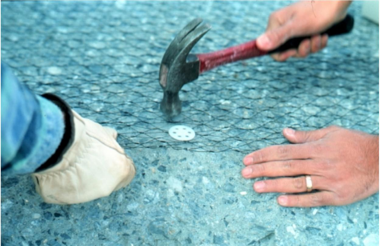
**Figure 2. Securing an activated titanium mesh on the concrete decks with plastic fasteners.**
