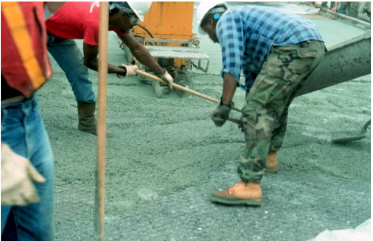
**Figure 5. Placement of a latex-modified concrete overlay over the deck, after the installation of the titanium mesh anode.**
