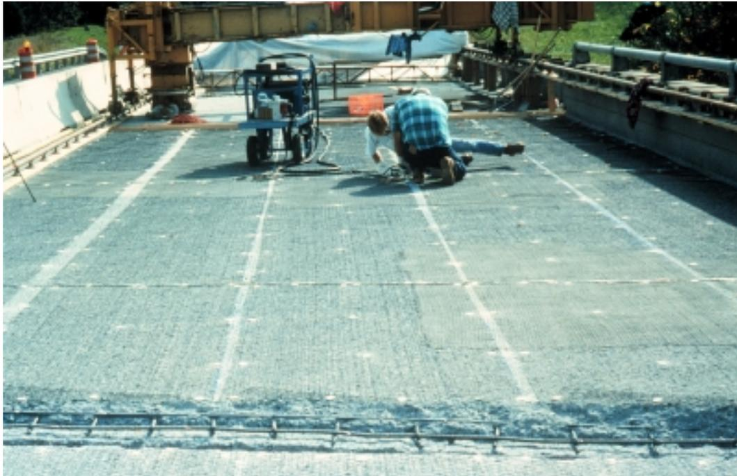
**Figure 4. For redundancy, additional titanium ribbons were welded transversely across the deck to all sections of mesh. Notice that the mesh sections were hardly distinguishable from the concrete deck surface underneath.**
