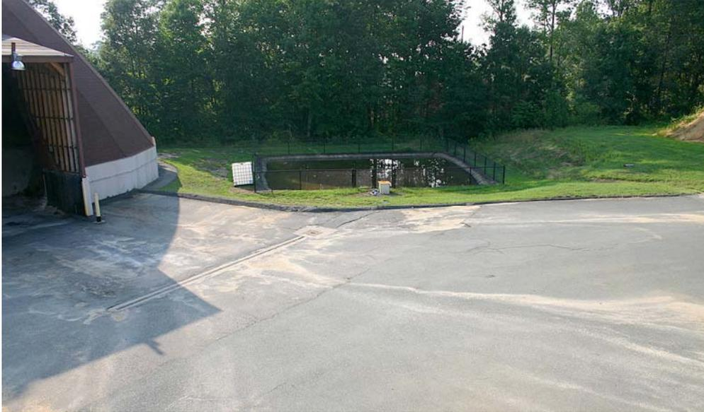
**Figure 1. Typical Salt Storage Structure, Loading Pad, and Stormwater Runoff Collection Pond**
