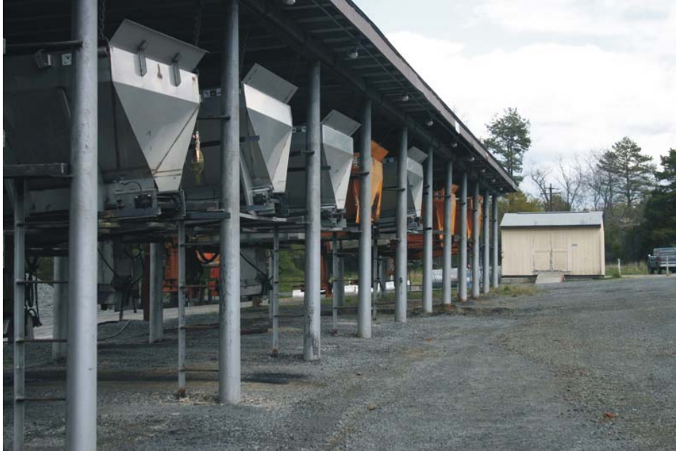
Figure 1. Salt-Spreader Racks Typical of Those Found at VDOT Area Headquarters Maintenance Facilities
