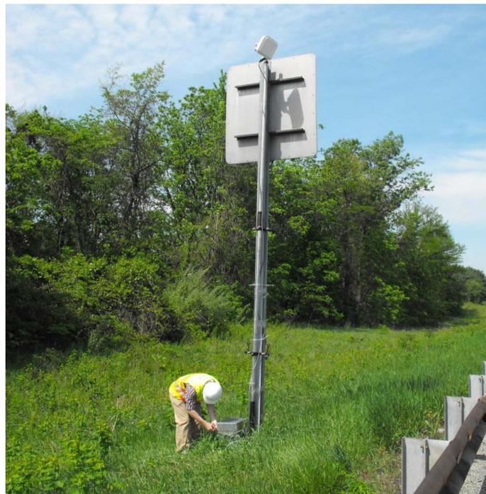
**Figure 2. Setup of Wavetronix Device Along I-81**
