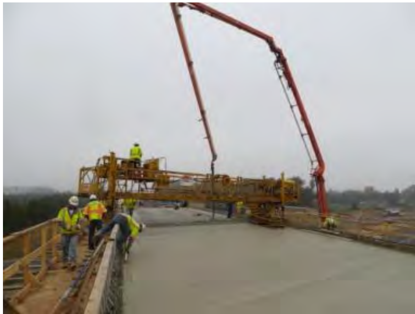
Figure 1. Concrete Placement and Screeding
