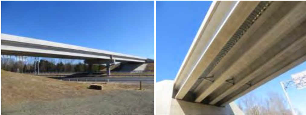
Figure 5. Bridge Beams With Lightweight Self-Consolidating Concrete
