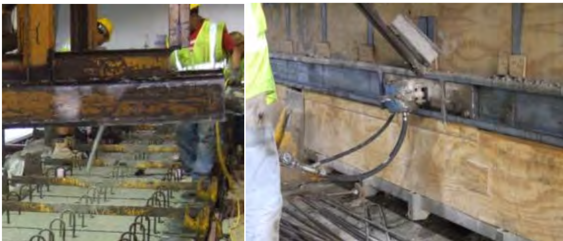
Figure 4. Internal and External Vibration of Self-Consolidating Concrete
