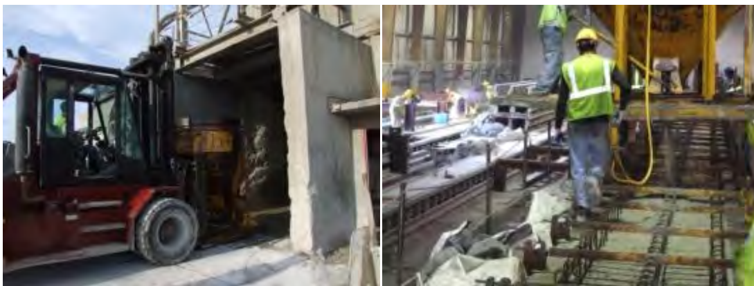
Figure 3. Placement of Self-Consolidating Concrete Into Beam Molds
