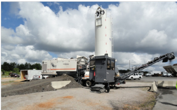
On-site mobile plant mixes reclaimed asphalt in cold central-plant recycling process.
