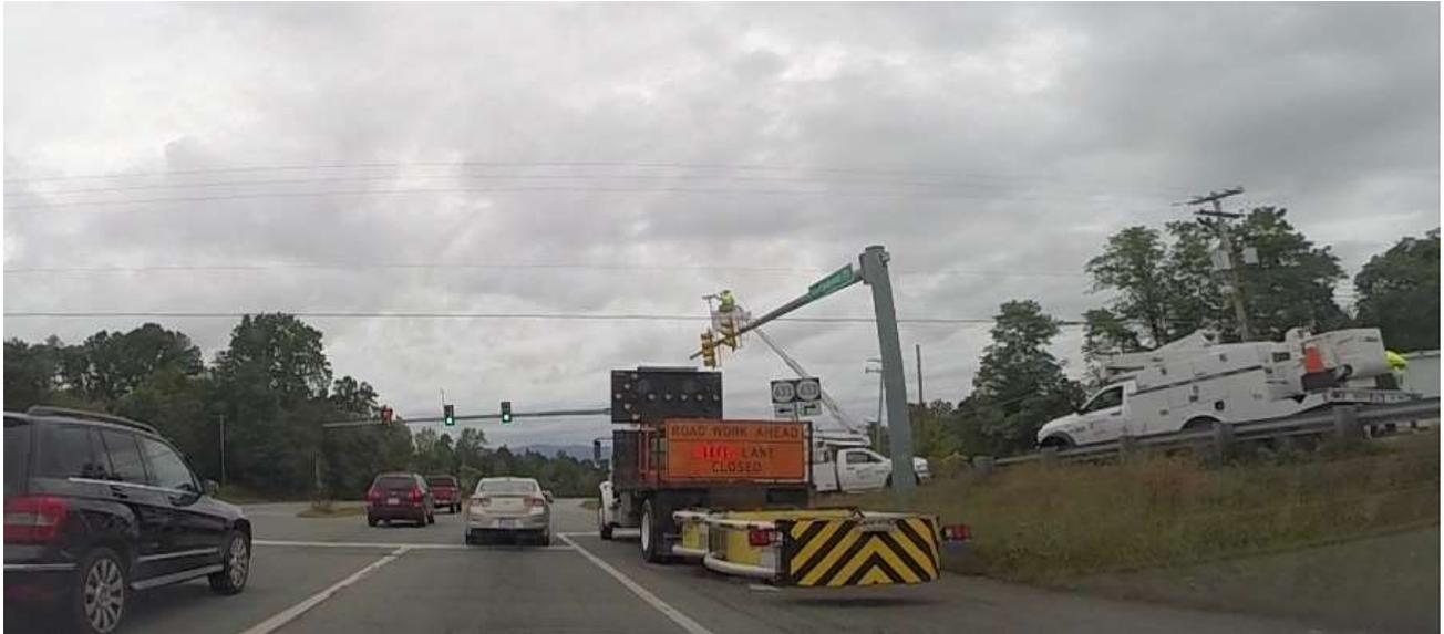
**Figure 32. Shadow Vehicle With Signing Error**
