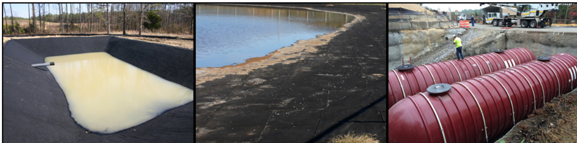
Figure 1. The Three Stormwater Storage Options Considered: New Ponds, New Liners, and Underground Storage Tanks
