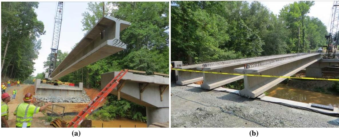
**Figure 4. Bridge Construction: (a) beams being delivered to the jobsite and erection of first beam; (b) three beams in place**
