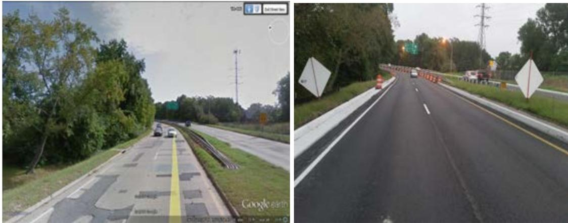
**Figure 14. Project Site Before and After Paving**
