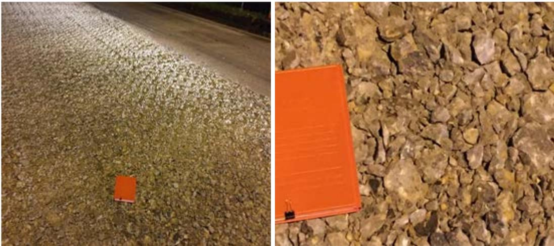
**Figure 11. Final Rubblization Surface**
