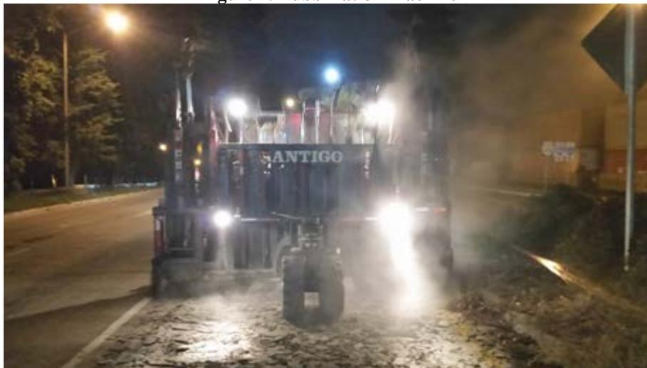
**Figure 5. Rubblization Process**
