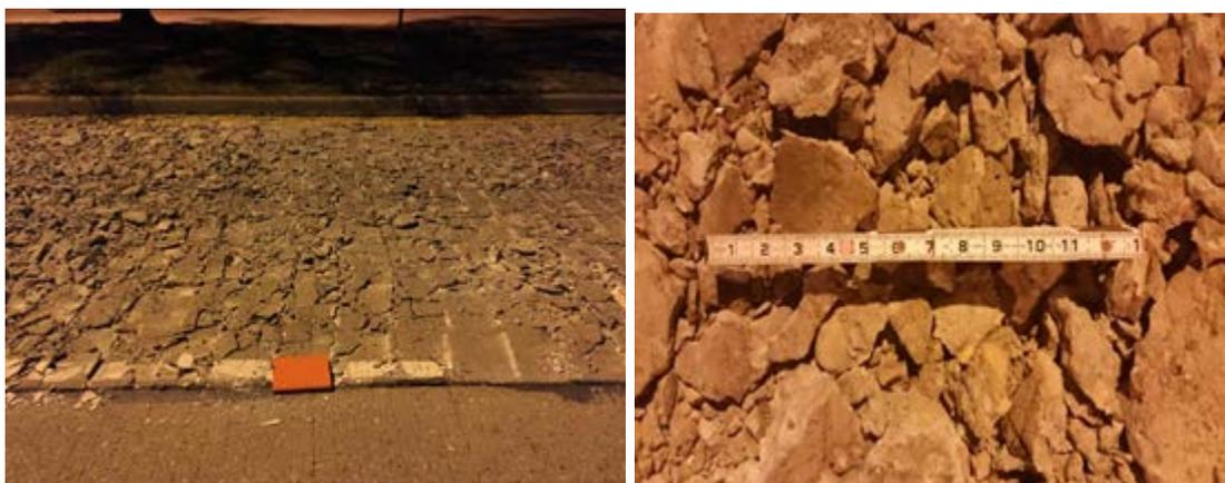
**Figure 6. Particle Size After Rubblization (Before Rolling)**
