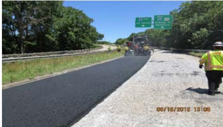
**Figure 12. Placement of IM 19.0E Mixture**
