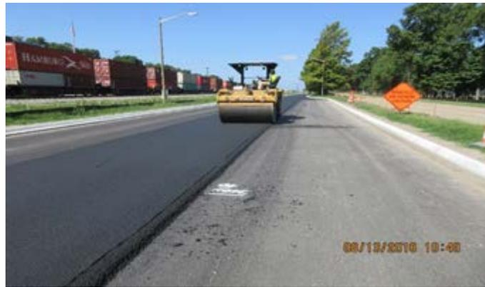
**Figure 13. Placement of SM 12.5E Mixture**
